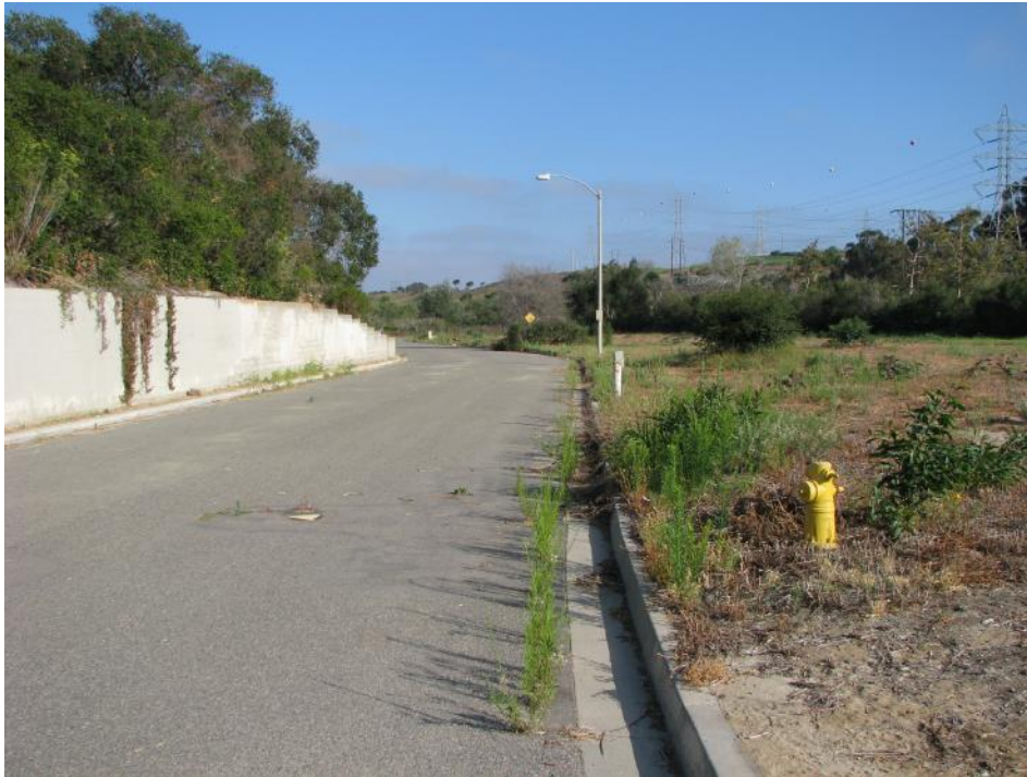
9. View to northwest of Site.
