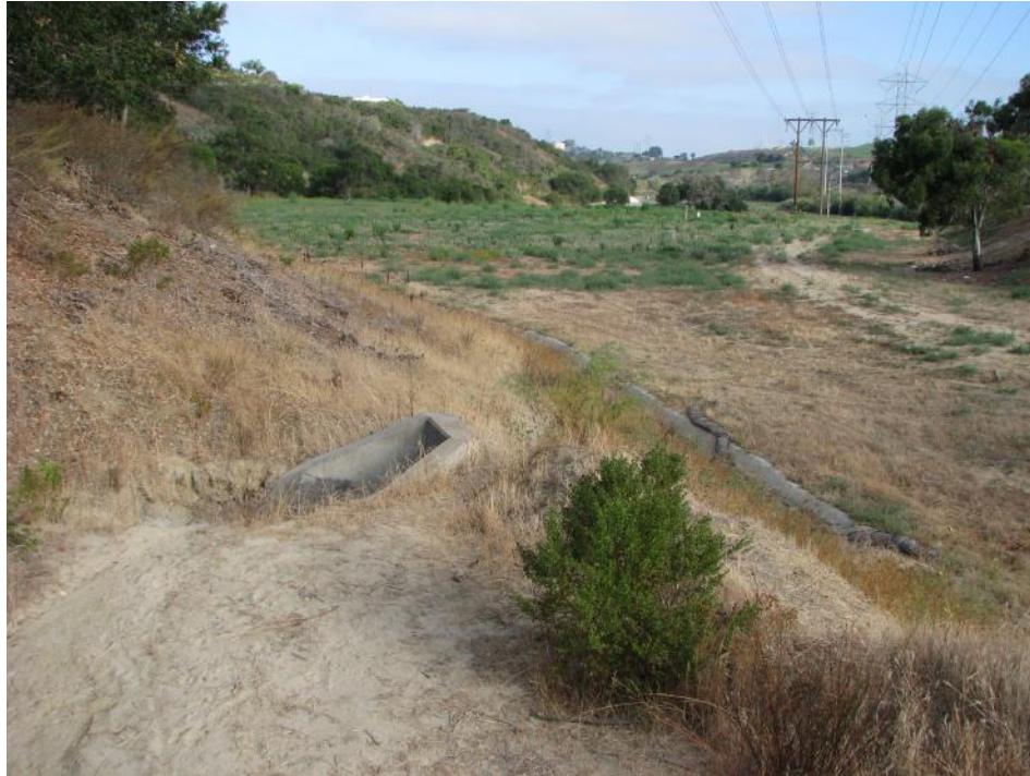
1. View to northwest of Site.
