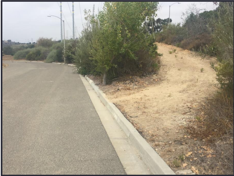
Photograph 13. View to the east at existing SDG&E easement road that will be improved and designated for emergency secondary access.
