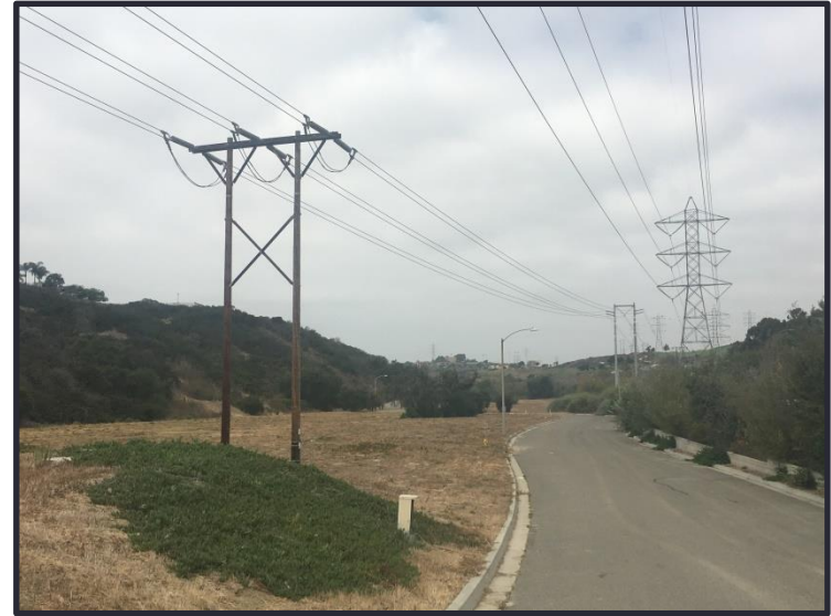
Photograph 10. View along existing West Oaks Way at electrical transmission lines, lighting, and hydrants.
