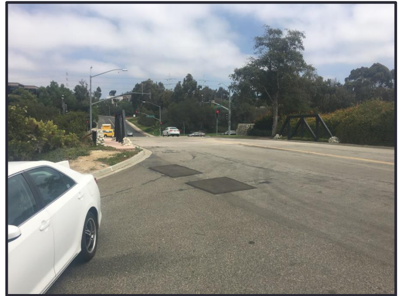
Photograph 2. View to the north along Palomar Oaks Way. Road is 52 feet wide and includes a left turn lane on northbound side.
