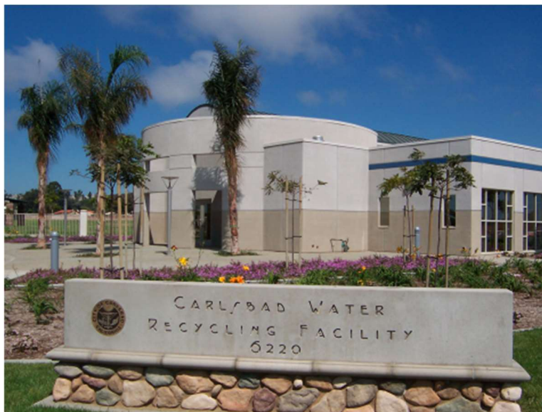
Carlsbad Recycled Water Facility (Carlsbad WRF)
