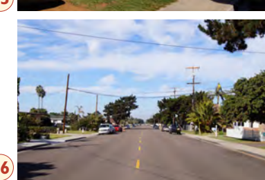
Most roads are wide, without consistent street trees and some with utility poles overhead.
