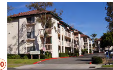
Housing density varies from single family homes to higher density structures such as this apartment building.
