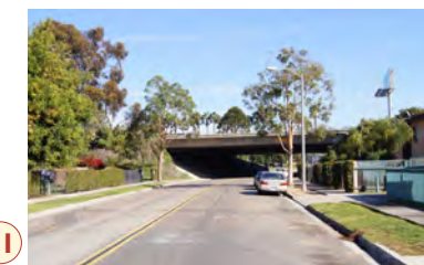
Freeway underpass at Chestnut Avenue
