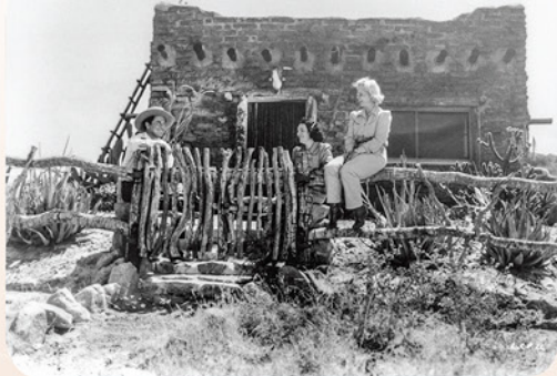
Leo, Deedie and Tony Carrillo circa 1940. In Pueblo architecture, a flat roof is traditional. Vigas , or rounded roof beams, extend through walls to the exterior. The horno , or oven, was modeled after the hornos of the southwest.
