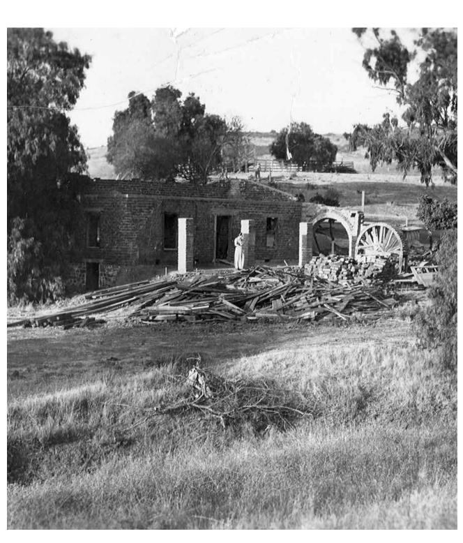
The second story was removed from the Kelly adobe house. See the wooden frame used to support the Spanish style arch during construction?
