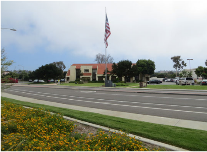
View of existing on-site commercial (office) building.
