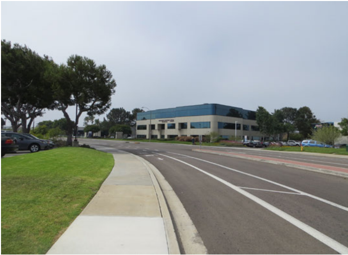
Avenida Encinas and commercial uses associated with the Pacific View Plaza to the southwest of the project site.
