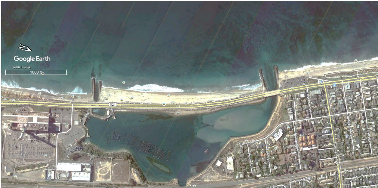
Figure 2-15. Agua Hedionda Jetties (Google Earth, 2021)
