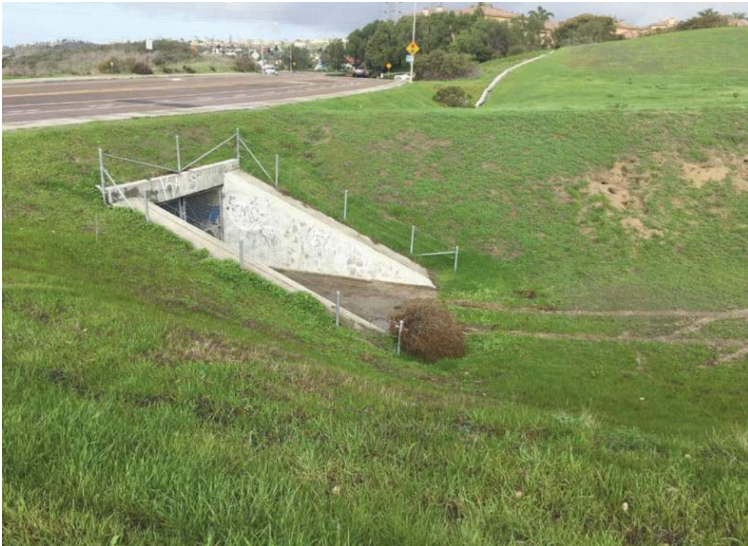
2) View of a drainage culvert located at the Site.
