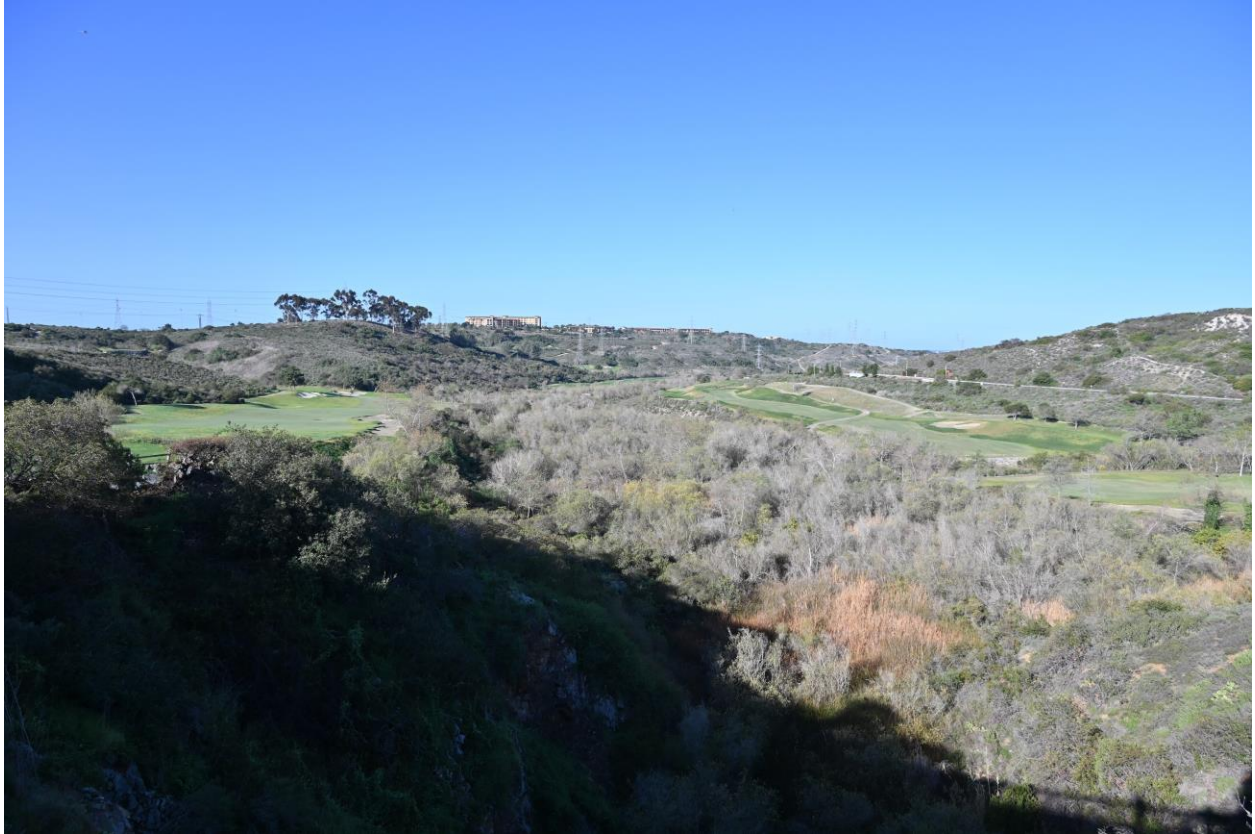
From Channel Upstream Begin Point - Looking Downstream at Natural Channel Below Project
